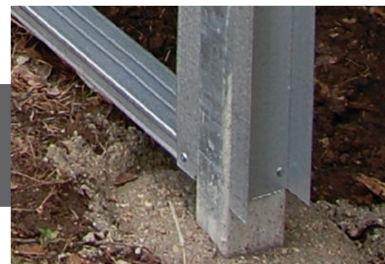
24 GA Track fastens vertically to 16 GA posts on both interior sides of 24 GA horizontal studs
