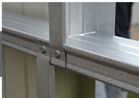
Detailed view of prefabricated vertical blocking members attached to horizontal metal studs
