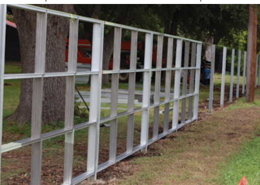
Fence structure made from 24 GA Spaceframe components and 16 GA Cee-Channel posts
