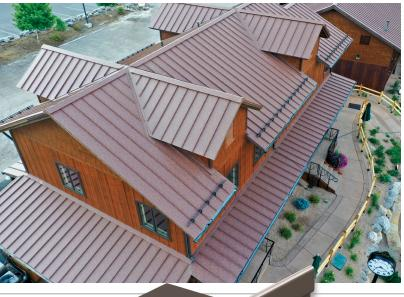
The Berridge Cee-Lock Panel is an architectural metal standing seam panel that incorporates an integral snap-lock seam and an optional patented vinyl weatherseal.
