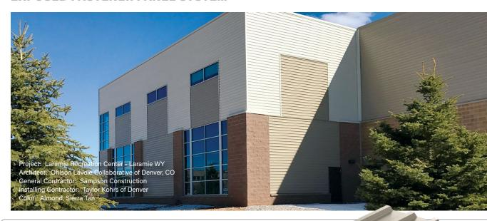
The Berridge "M" Panel is a wide, economical panel providing 36" of coverage for vertical and horizontal applications with exposed fasteners.
